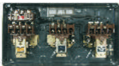
Interior View of MK2 FASD
