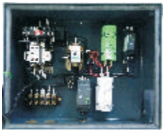
Interior View of MR-G2W
